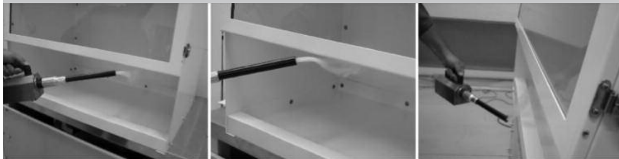
FIGURE 30. AIRFLOW SMOKE TEST – EXTERNAL PERIMETER
